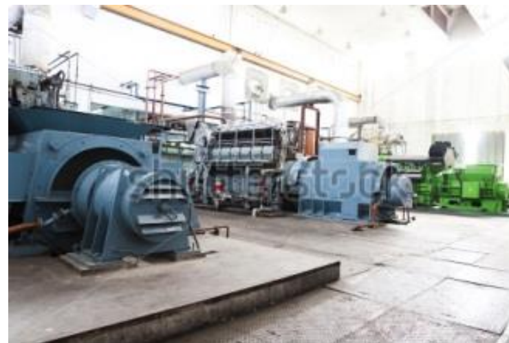
Diesel backup generator
