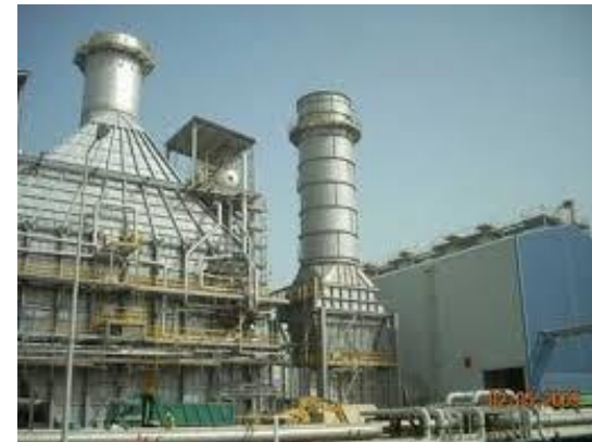
Combined Heat-Power Plant (CHP)
